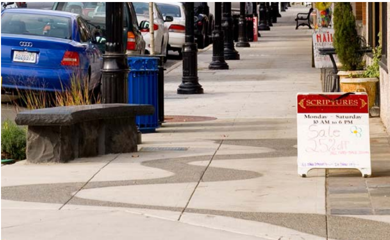
Sandblast Finish over Sidewalk
