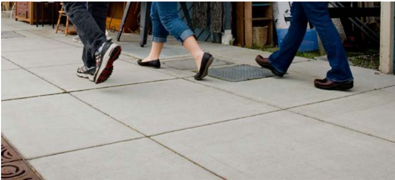
Sidewalk with 2'x2' Sawcut Scoring
