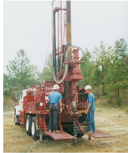
Truck mounted drill rig.
